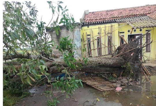
Figure 3. Residents' Houses in Kohod Village, Pakuhaji District Collapsed After Being Hit by Strong Winds 26 / 02/2021
