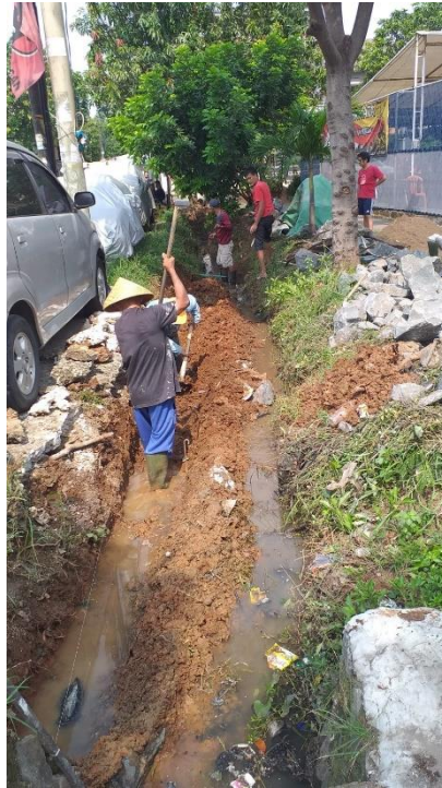
Figure 7. Soil excavation.
