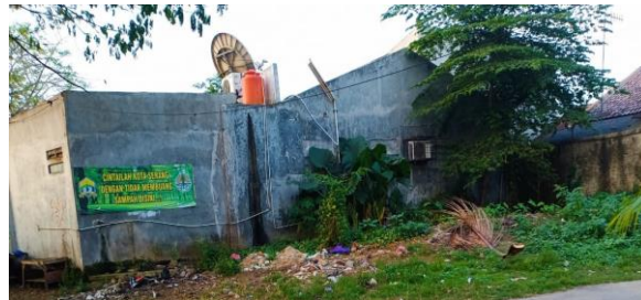
Figure 2. Vacant Land Before Cleaning
