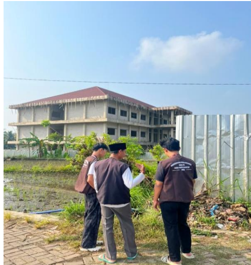
Figure 1. The implementation team conducted a location survey in Panday Village, Batubantar Village.
