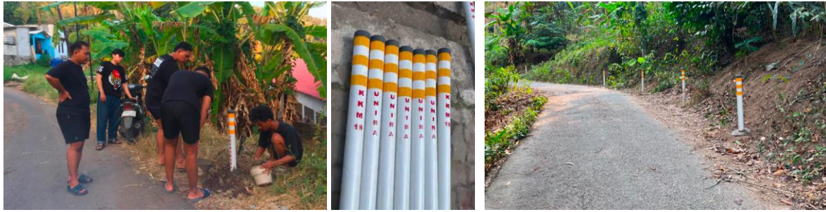
Figure 3. Implementation of the Manufacture and Installation of Road Reflectors
