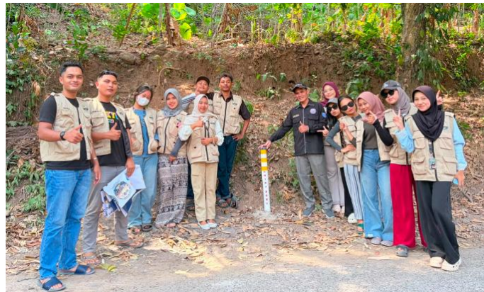
Figure 2. Activity Planning and Sample Street Lighting Installation
