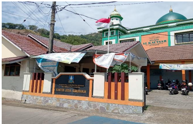
Figure 1. Sumuranja Village Office
