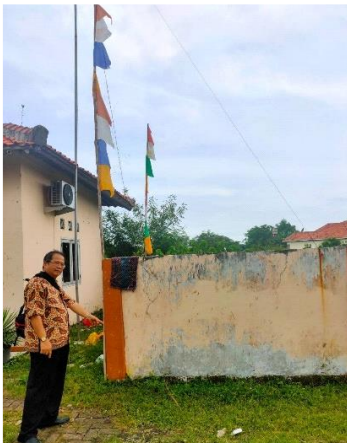
Figure 2. Poor Drainage Figure
